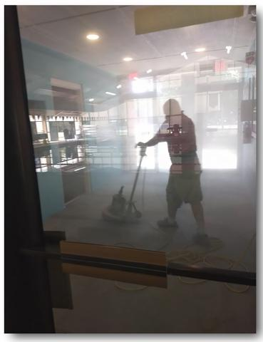
It's not as simple as just putting down new paint and sealant. All floors required sanding, washing, painting, sealing and texture.
