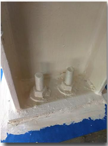
Steel beams on the pool deck at Bluffton Pool had heavy oxidation. Staff washed, sanded, washed again, and painted over three dozen of these throughout all three indoor pools while pools were closed to the public.
